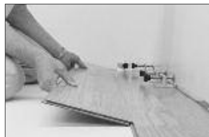
Begin second row with at least 12" stagger of end joints, assemble the first panel in the second row to the adjacent panel in the first row by slightly angling tongue into groove until plank locks into position. Insert the tongue at about a 20° angle and lock the planks together. (Use non-marring blue tape to secure the panel across the assembled joint to hold it in place.)
