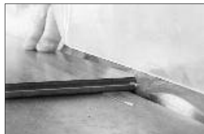
Cut off all milled profiles from the edges abutting vertical surfaces. This provides a solid edge to receive spacing devices.
